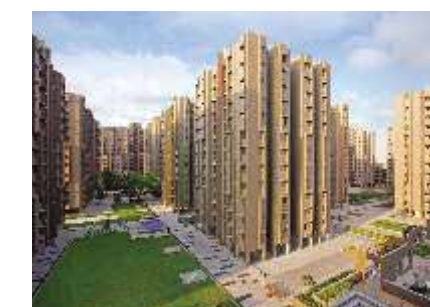
2 & 3 BHK Apartments at Khokhra, Maninagar, Ahmedabad
