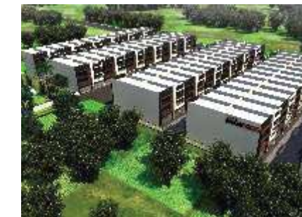
Industrial Sheds on Naroda Road, Ahmedabad
